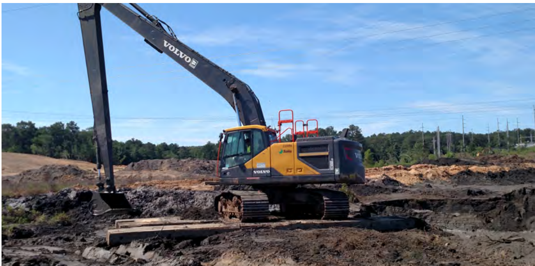
EXCAVATOR WORKING SAFELY FROM SWAMP MATS
